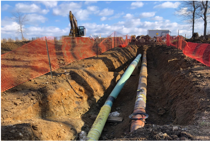
Mariner East, 12" interconnect in Middletown, PA. Photo taken by Eve Miari
